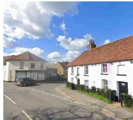
ROYDON: Harlow Road (source: Google Earth Pro)
