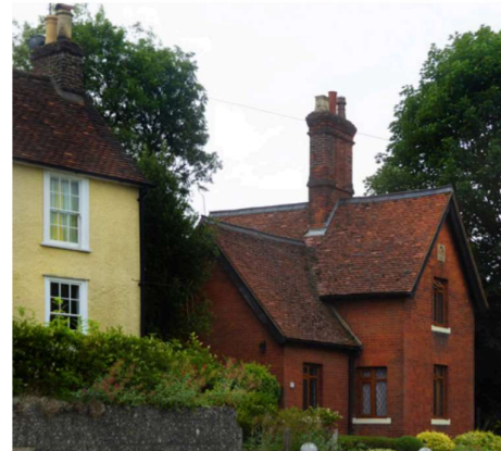
PYE CORNER: distinct tall decorative chimneys and gables with windows (source: GANP)
