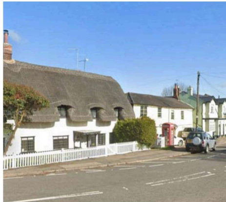
WIDFORD: variety of 2 storey built form with the characteristic white render (source: Google Earth Pro)
